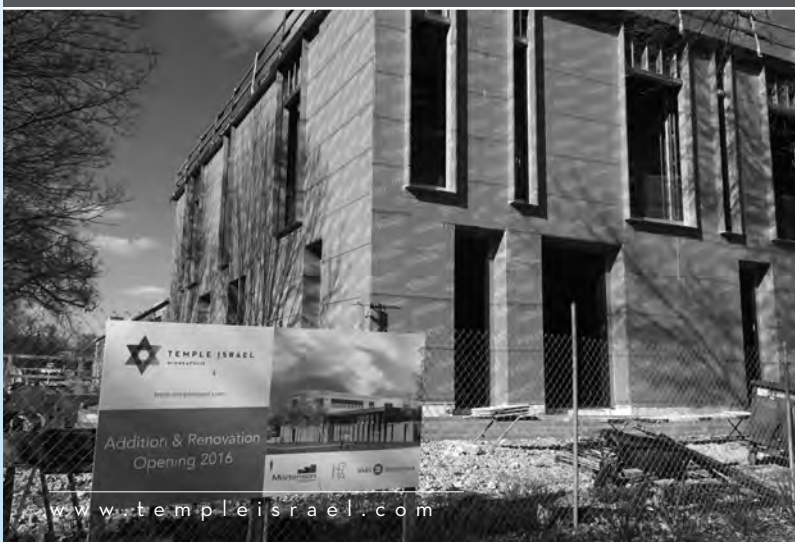
Project sign and southwest corner
